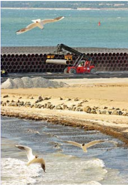
Storage and loading of pipe joints for the Nord Stream gas pipeline on the German Baltic Sea coast.
