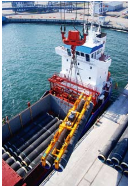
Storage and loading of pipe joints for the Nord Stream gas pipeline on the German Baltic Sea coast.
