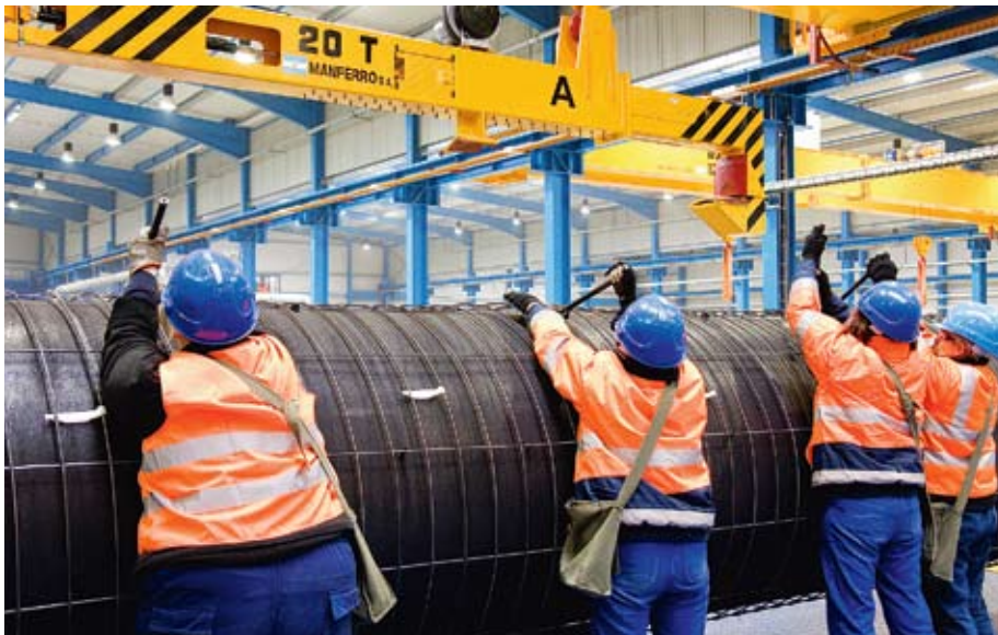
Workers installing equipment for the Nord Stream gas pipeline that will link Russia and the European Union via the Baltic Sea.
